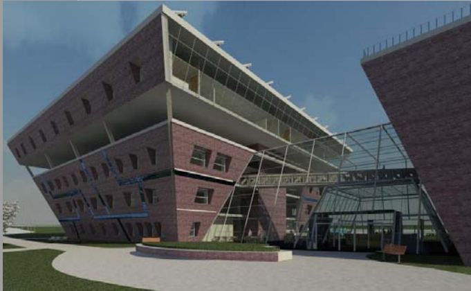
View of Tower and Atrium
